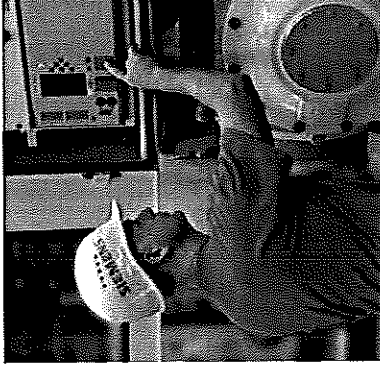
Bay control systems in ergonomically arranged local control cabinet
