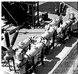
Outdoor GIS 8DN8 (HIS switchgear, 5-circuit-breaker H-arrangement).
